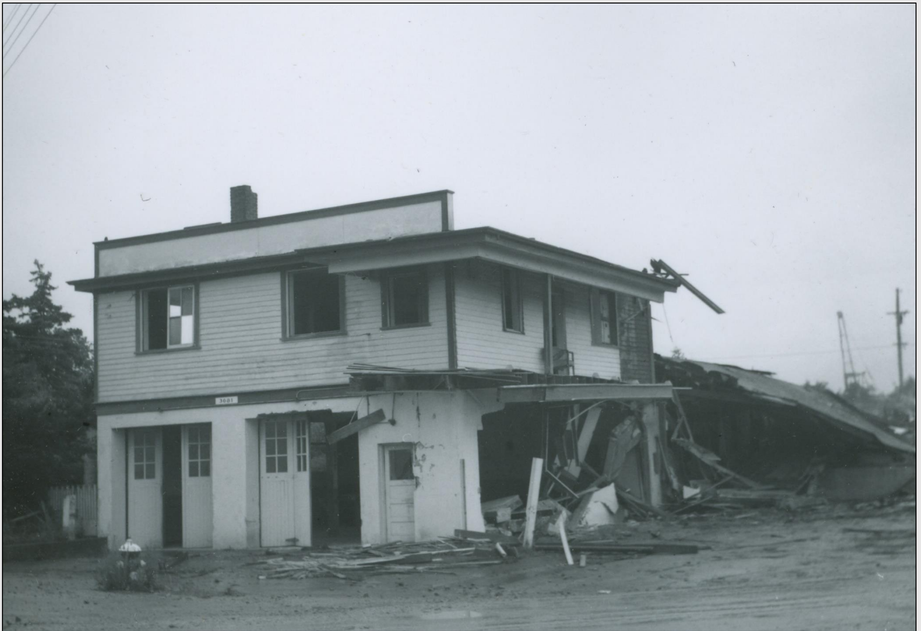
Demolition of No. 1 Fire Hall, 3681 Douglas Street, 1964 (1980-015-094a)
